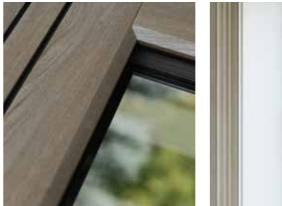
In the UK where external shutters are rare, the vast majority of casements open outwards. Within casements, there are various styles. A flush casement is simply one where the opening window sits flush in its frame, rather than standing proud.
