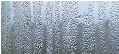
Condensation on interior face of a DGU
